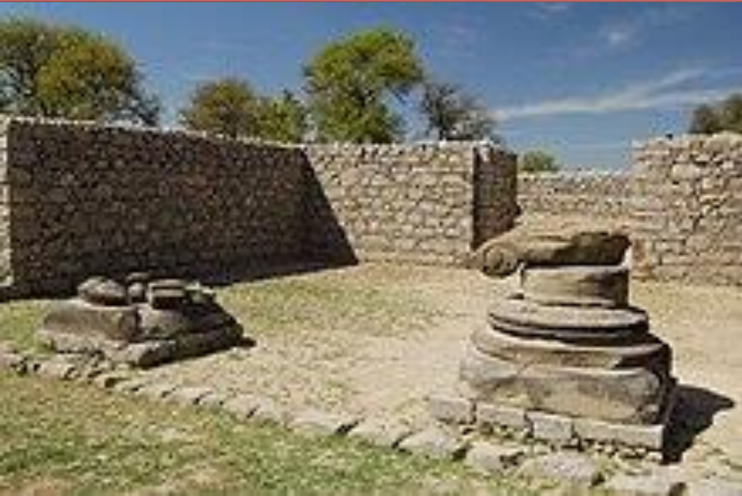
The Hellenistic temple with Ionic columns at Jandial , Taxila , Khyber Pakhtunkhwa , Pakistan . It is usually interpreted as a Zoroastrian fire temple from the period of the Indo-Parthians.
